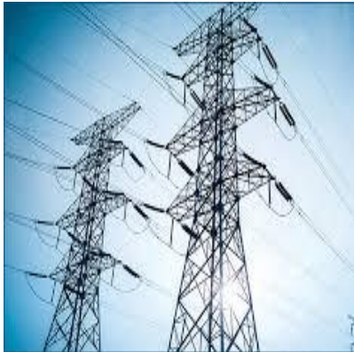
Electric power T&D
